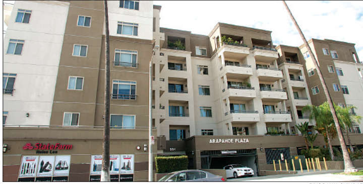
Checked In: Retail-condominium property Arapahoe Plaza in Koreatown.
